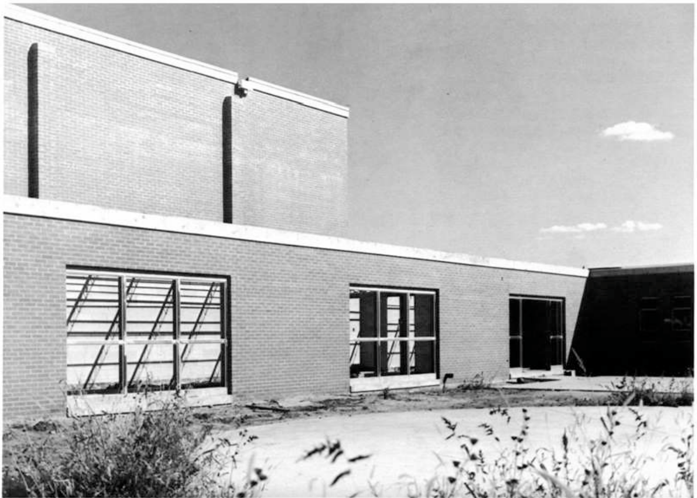
The proposed Senior Court as it appeared under construction.
