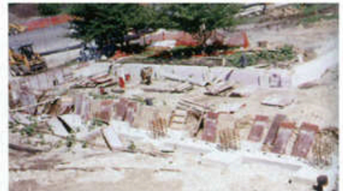
▲ An aerial view shows the extent of construction.
