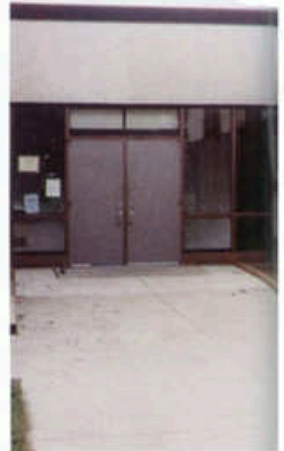
▲ This is Lisle's temporary entrance.
